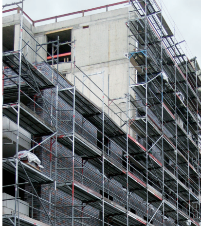
Pipe coupler scaffolding
