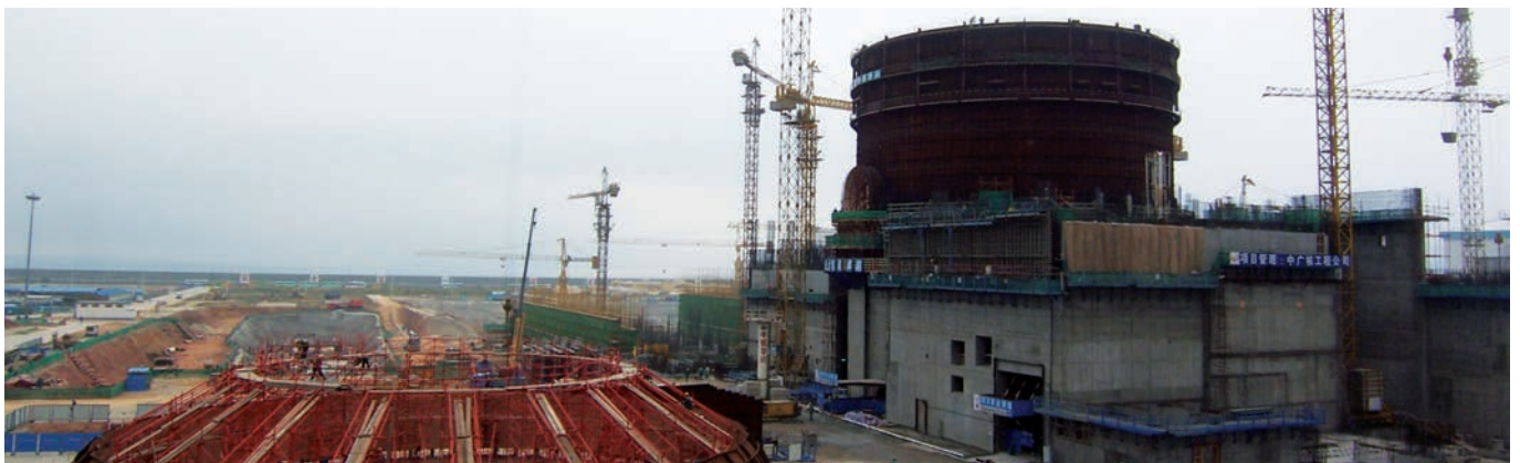
Nuclear power plant under construction
