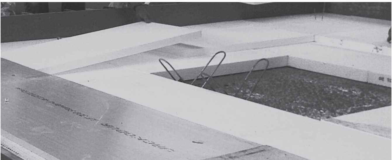
Installation of SP-SPA-2 at a precast plant.
