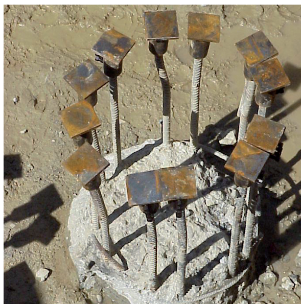
End zone detail in one pile
