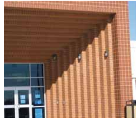
Custom Designed Corbelled entry.
