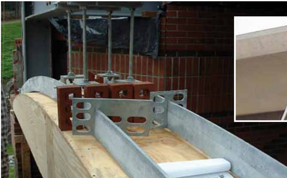
Mid spans connected to embeds in concrete.
