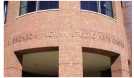
Custom Designed Planned Radius Brick Soffit.
