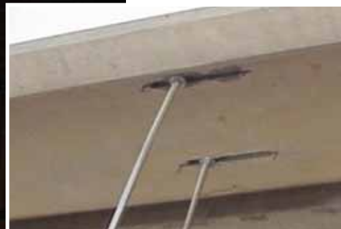
Mid spans connected to embeds in concrete.
