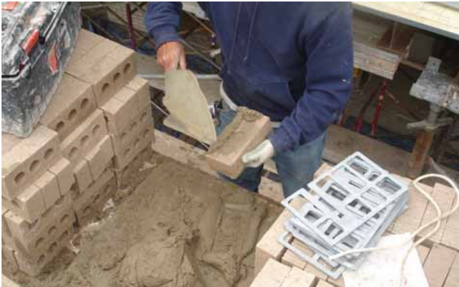
Fill cored brick with mortar.
