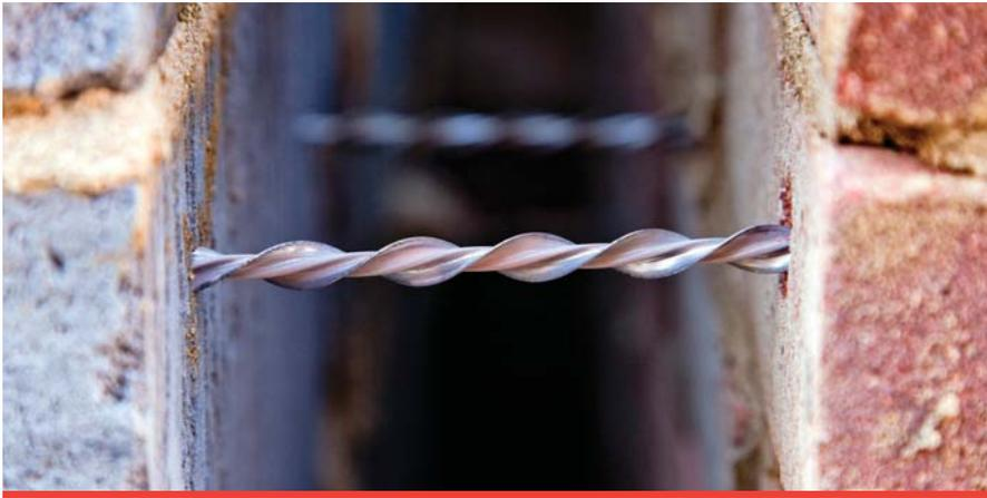
Helifix remedial wall ties can be installed to connect outer wythe masonry façades to inner wythe masonry walls or structural frames, roof and floor joists. Depending on application details, remedial wall ties may be installed into clearance holes with HeliBond cementitious grout, with epoxy resin or driven into position to provide a dry, mechanical connection.
