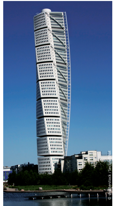
Turning Torso in Malmö (Sweden)
